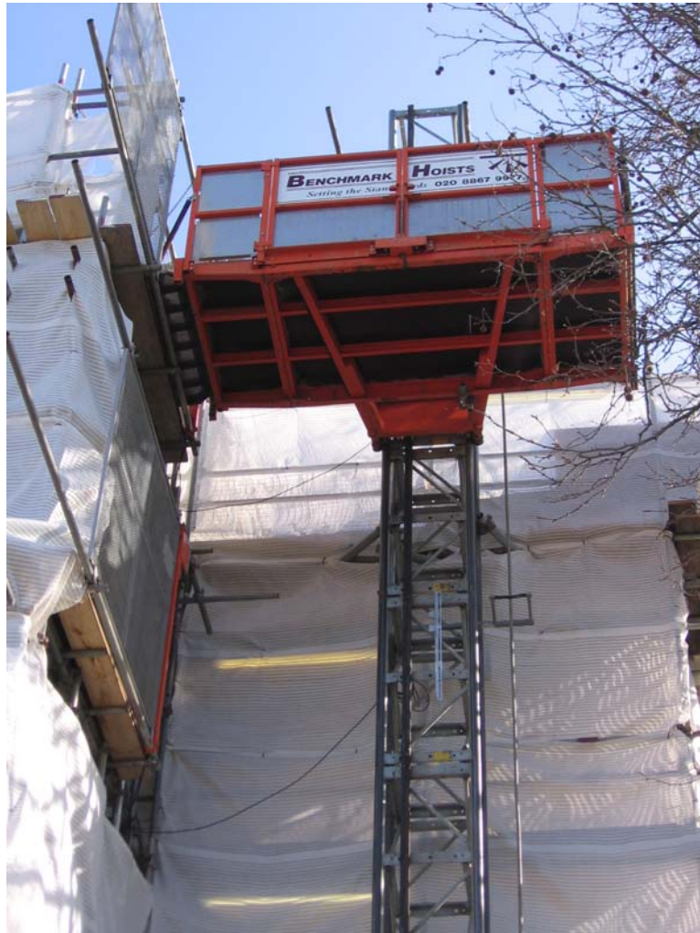
Photo 1 - M15/32 Goods Hoist – Bovis Lend Lease National Maritime Museum Greenwich
