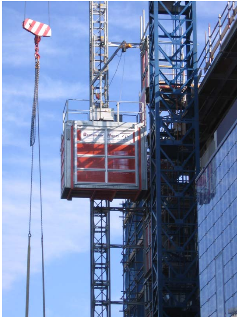
Photo 1 - Alimak 650 23/32FC Driverless Passenger/Goods Hoist
