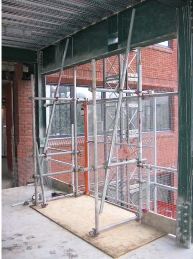
Photo 2 - Hoist Landing Gates & Hoistway Protection fixed to floors
