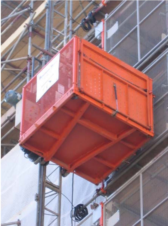
Photo 2 - M700 Goods Hoist showing C door for side loading at base level
