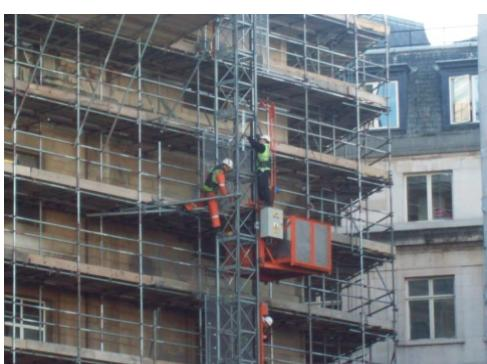
A milestone for **Benchmark** at the Café Royal was the installation of our first hoist. This was erected for Erith Demolition to aid the removal of asbestos from the building and was situated on the corner of Glasshouse Street by Air Street.
