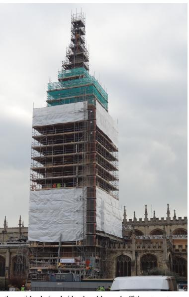
Only the south elevation is ground based with the other three sides being bridged and braced off the stone tower using a combination of 600 deep steel beams, 750 alloy beams & ladder beams.
