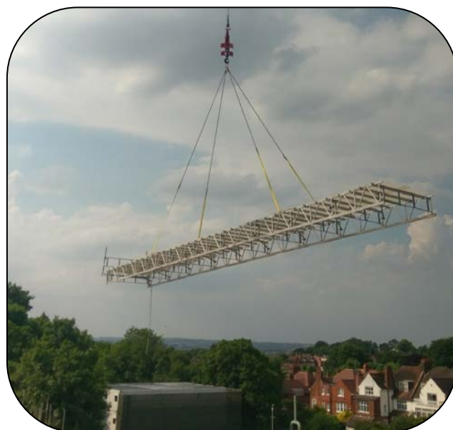
A roof section being lifted by the site crane.
