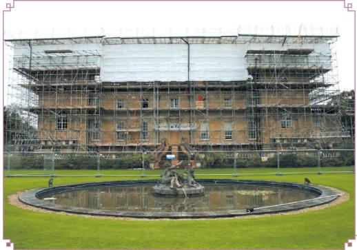
The scaffold structure which measures 48m long x 30m wide x 21m high is free standing because of the condition of the existing building and has been constructed using traditional tube and fittings with a Hakitec 750 panel roof providing weather protection.
